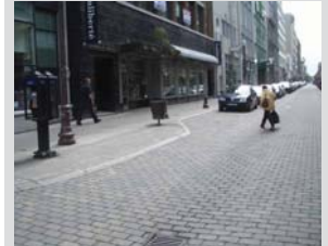
Street with rolling curbs
