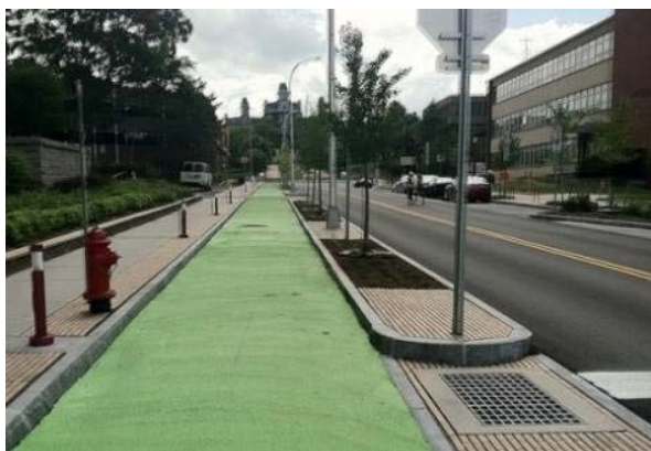
Concrete median islands with trees and light posts (Syracuse NY)
